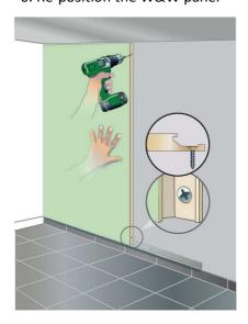
Attach the W&W panel with three BerryAlloc screws or use alternatively a nail gun.
